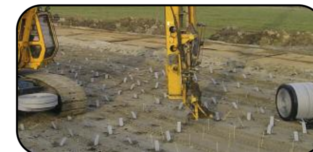
Thanks to its high performance Colbondrain is often the chosen PVD for major, technically demanding projects, such as the third runway at Changi Airport, Singapore. In this project Colbondrain has been installed to depths of up to 50 meters. The project required a total of 60 million linear meters of PVD and is one of the largest vertical drain reclamation projects in the world.
